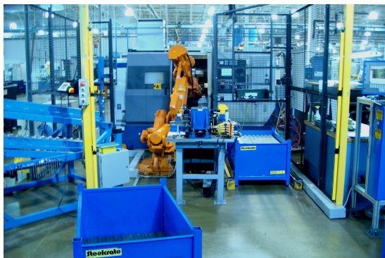
One of the cells from the part loading aisle
